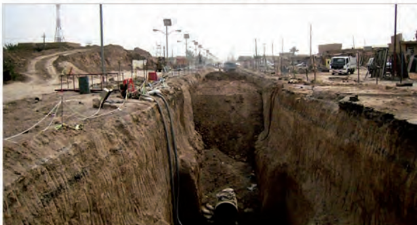
A wastewater treatment project in Falluja, Iraq, has tripled in cost to $100 million and is about three years behind schedule
